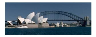
The construction of the Opera House is only possible because the distinctive shells come from a single geometric spherical section. This was not part of the napkin design — yet according to Utzorn, this "solves all the problems of practical construction by opening up mass production" both for the tiles on the roof, and the ribs supporting them. Without mass production of modular components the Opera House could not have been completed.
